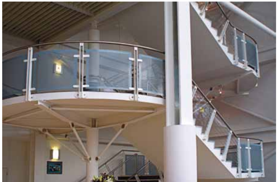
Balustrade infill panels with unperforated margins
